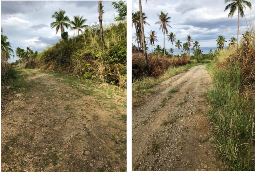
Portions of the Gumamela–Infres FMR, with concrete-paved portion on a critical slope
