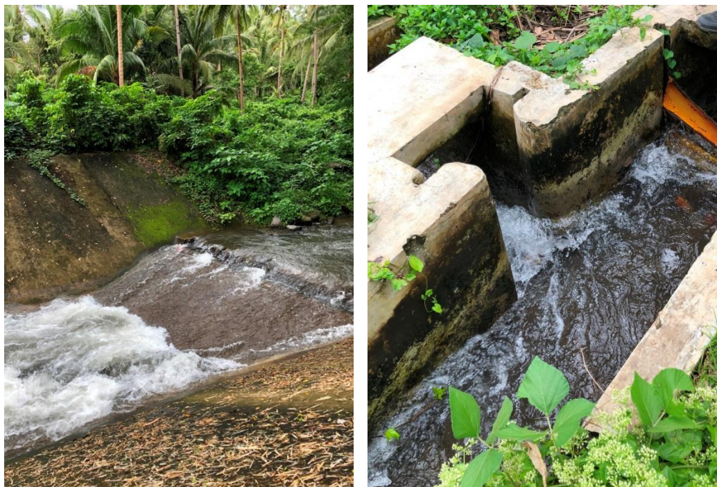
The main diversion structure (left) and one of the turnouts (right) of the Cabucgayan CIS
