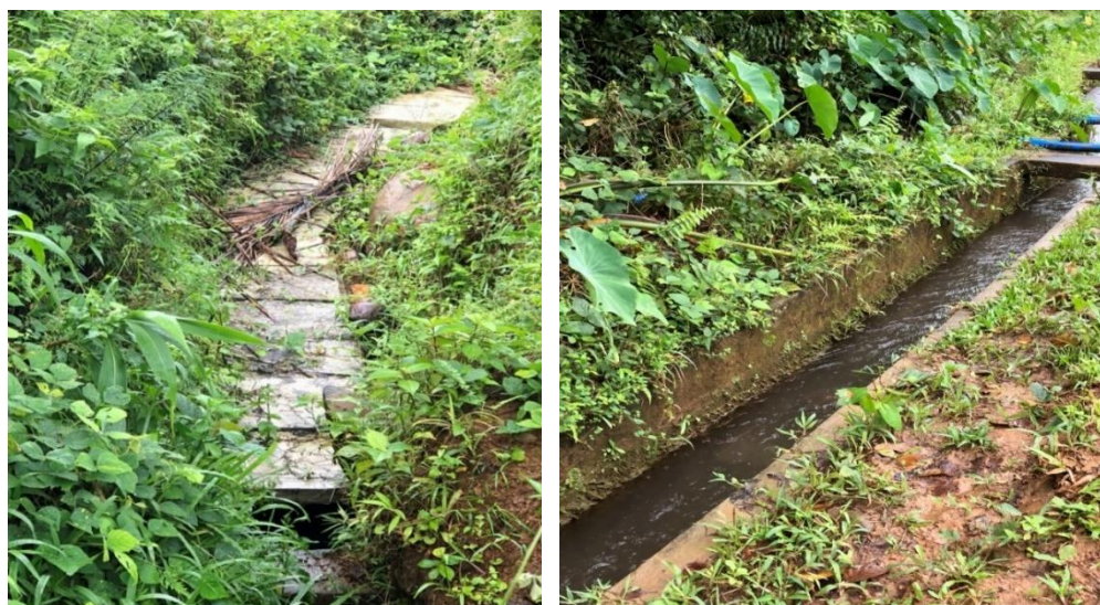
Portions of the main canal with concrete cover (left) and without cover (right)
