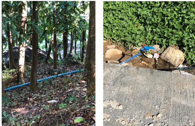
The main pipe from the reservoir (left) and an existing tap stand beside the road (right)
