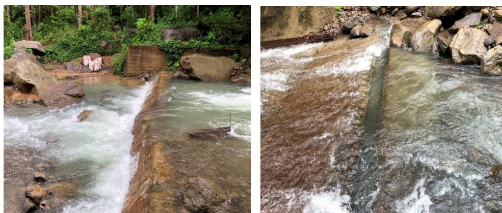
The downstream portion (left) and the upstream portion (right) of the main diversion structure
