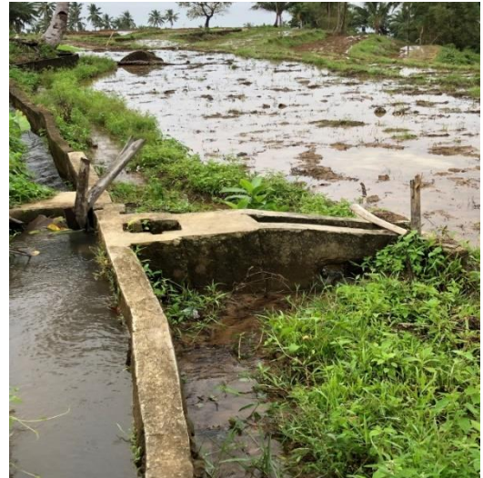
Some of the canal structures and turn-outs that were constructed
