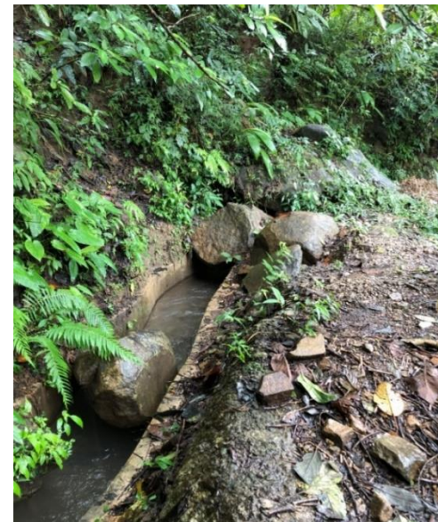
Portions of the canal that were destroyed by boulders during the landslide and Typhoon Urduja
