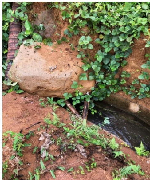
Portions of the canal that were destroyed by boulders during the landslide and Typhoon Urduja
