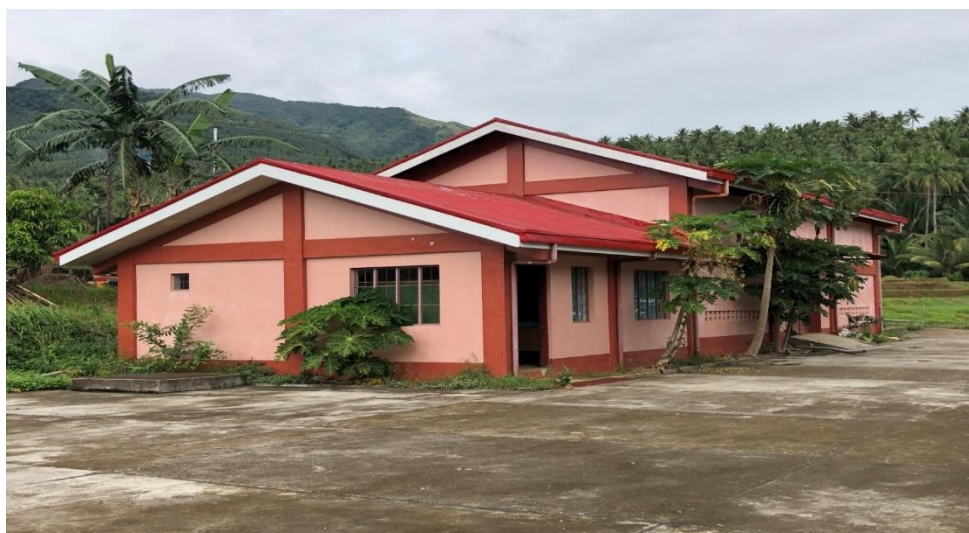
The Balaquid Post-Harvest Facility building and sun-drying pavement
