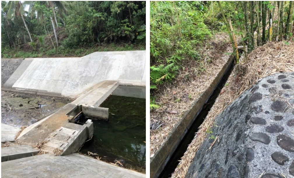
One of the dams (left) and a portion of the irrigation canal system (right) of the Hingatungan CIS
