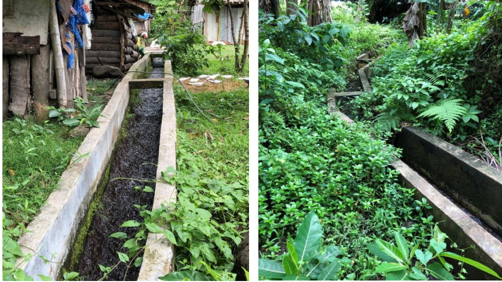
Portions of the concrete-lined canals of the Cabucgayan CIS
