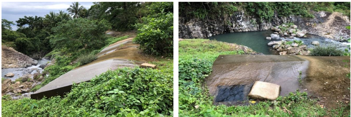
The main diversion structure of the Balaquid CIS
